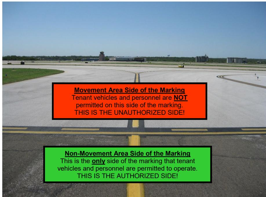
**Runway Holding Position Markings** are located across each taxiway that leads directly onto a runway. These markings are made up of **two solid lines** and **two broken yellow lines** and denote runway holding position markings. These markings are always co-located with a Runway Holding Position Sign. A vehicle operator must not cross from the solid-line side of the marking without first obtaining clearance from the FCT.
