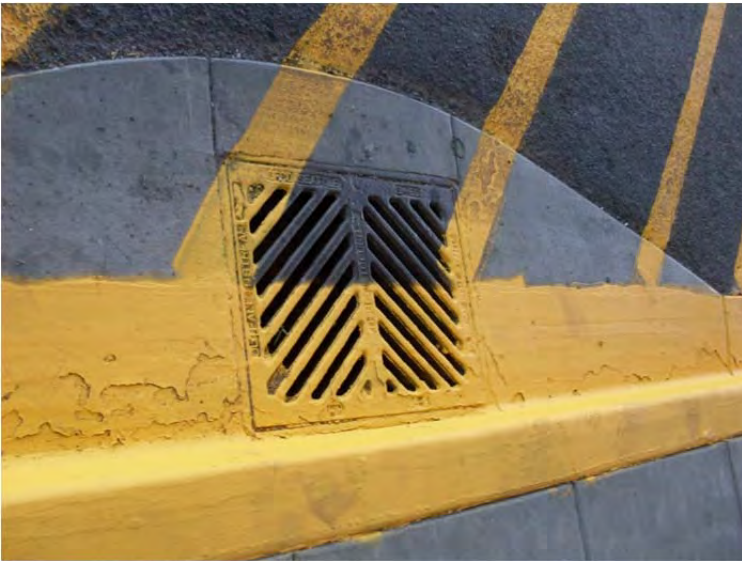
M-1: Storm drain catch basin at entry drive
