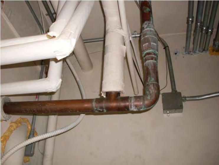
M-34: Missing domestic water pipe insulation
