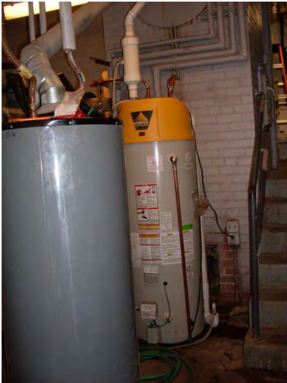
M-44: Newer 90% efficient condensing water heater
