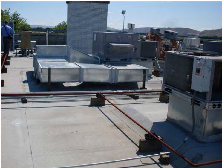
M-19: Galvanized steel rooftop ductwork
