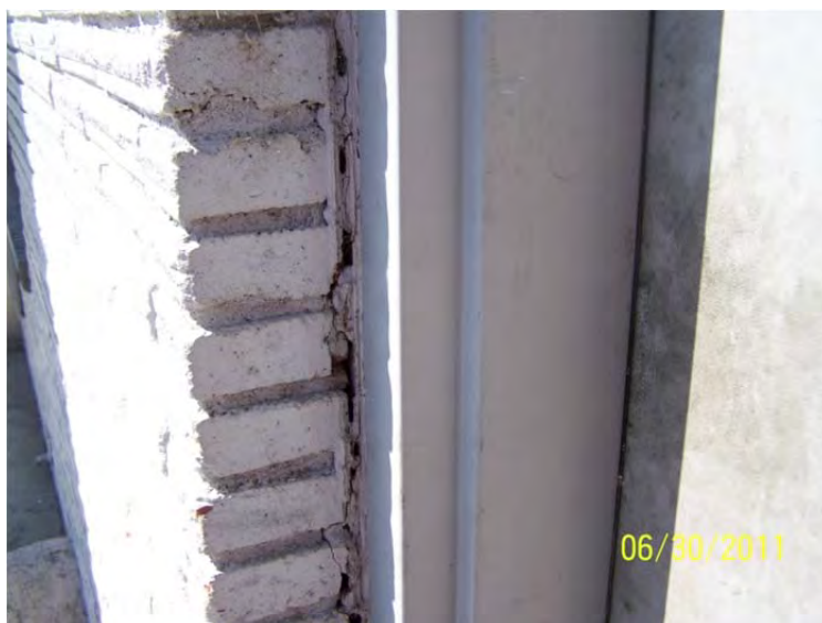
S-2: Deteriorated caulking at exterior face brick veneer
