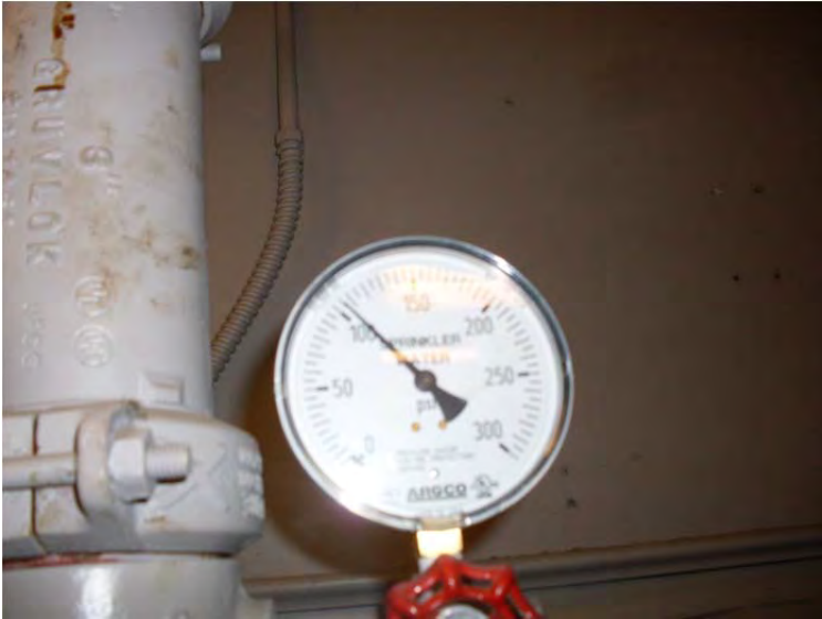
M-42: Fire water service pressure = 105 psi static
