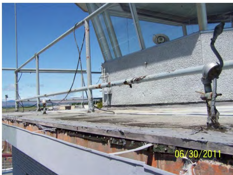
S-4: Roofing system and flashing in need of repair at low roof at former airport traffic control tower
