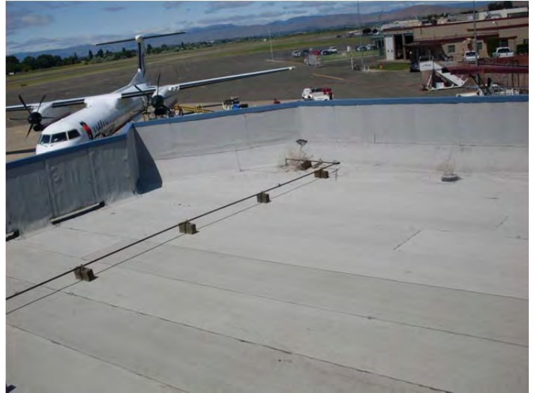
M-14: Rusty milled steel rooftop gas piping
