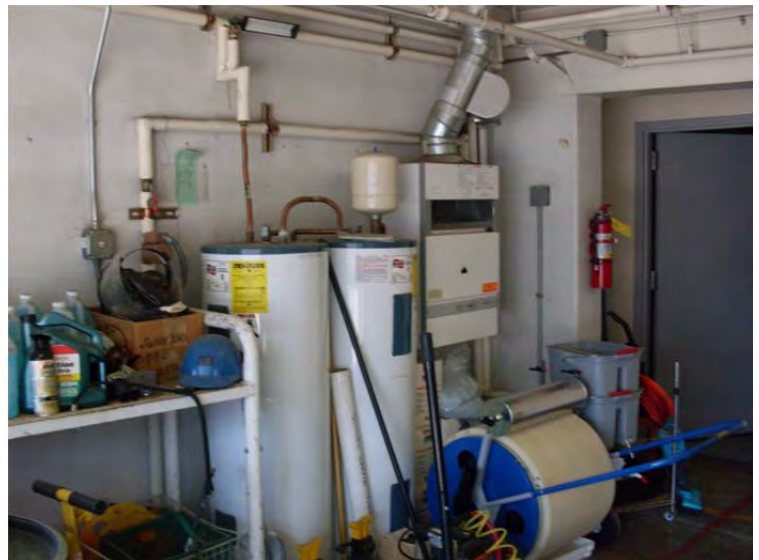
M-16: 80% efficient instantaneous gas water heater
