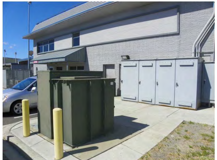
E-12: Transformer and main switchboard
