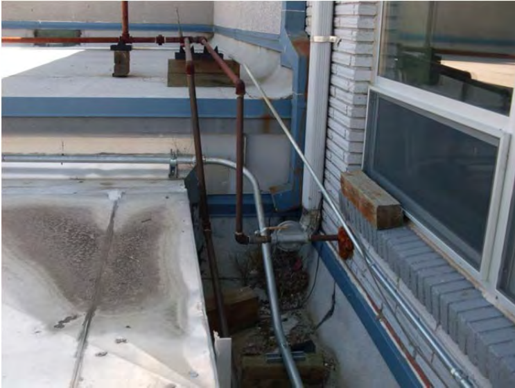
M-17: Rusty mild steel rooftop gas piping
