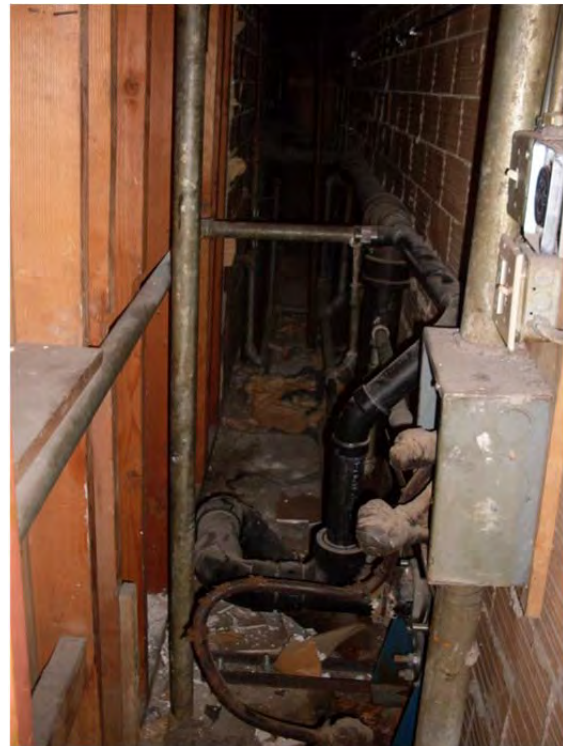
M-37: Plastic waste and vent piping repairs
