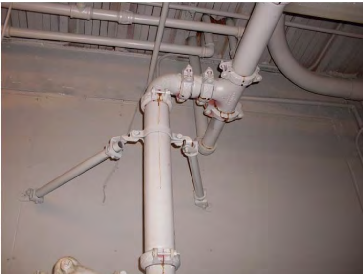
M-40: Fire sprinkler pipe with mechanical joints
