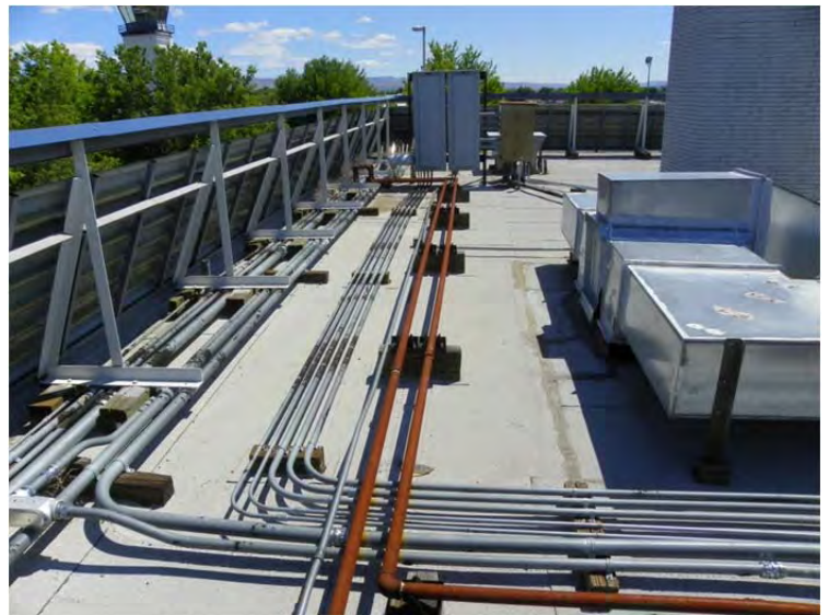
E-8: Roof panels and conduit routing
