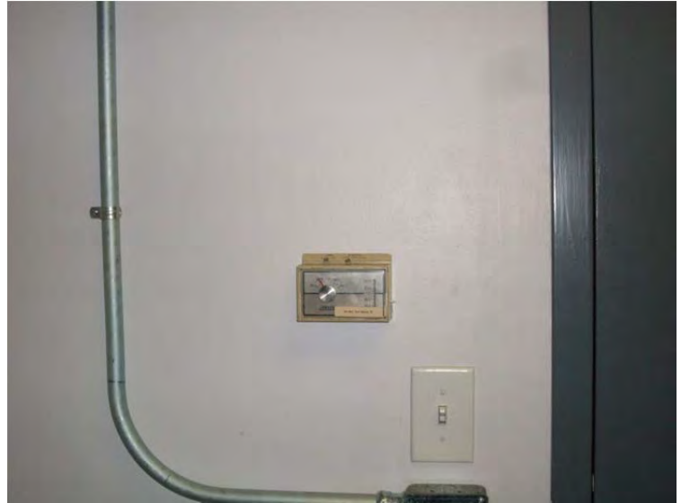
M-35: Typical wall mounted thermostat
