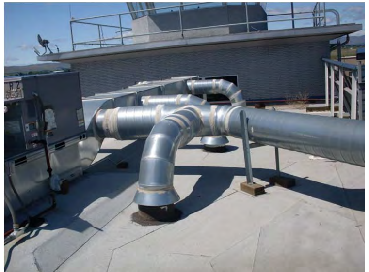
M-20: Double wall galvanized rooftop ductwork
