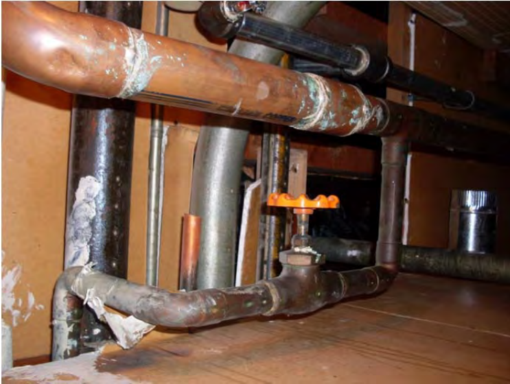
M-38: Copper domestic water with brass valves
