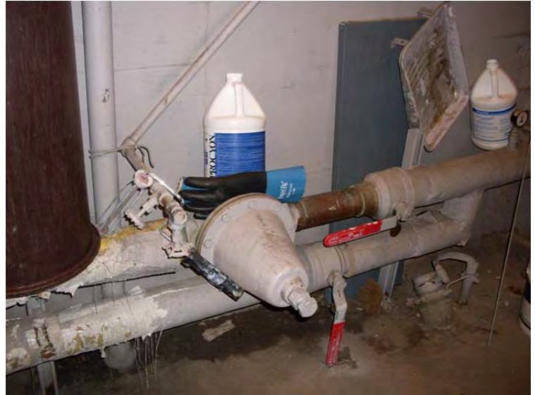
M-43: Main domestic water regulator without relief
