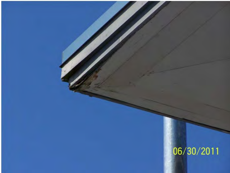
S-5: Water damage in fascia and overhanging soffit
