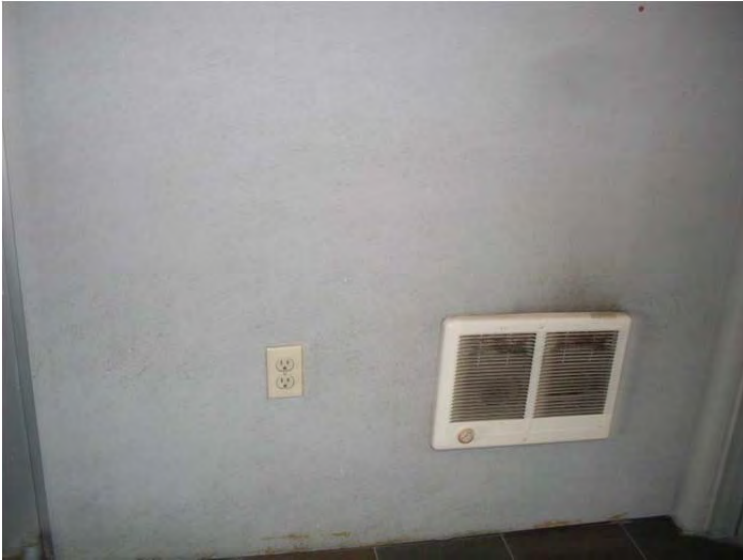
M-26: Typical wall heater
