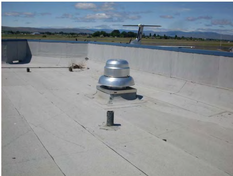
M-15: Aluminum mushroom roof exhaust fan
