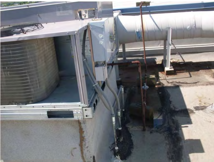
M-11: Split cooling unit condenser
