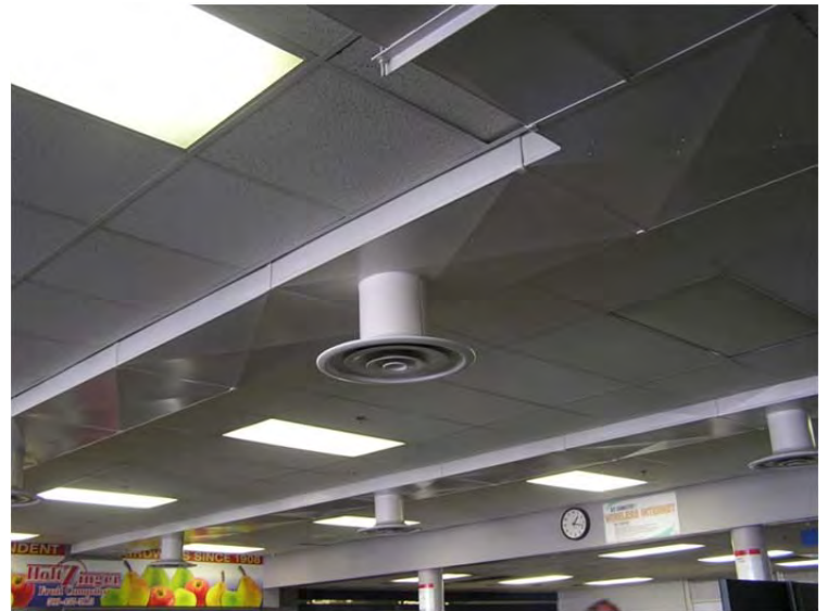
A-29: Exposed ductwork in ticket lobby ceiling
