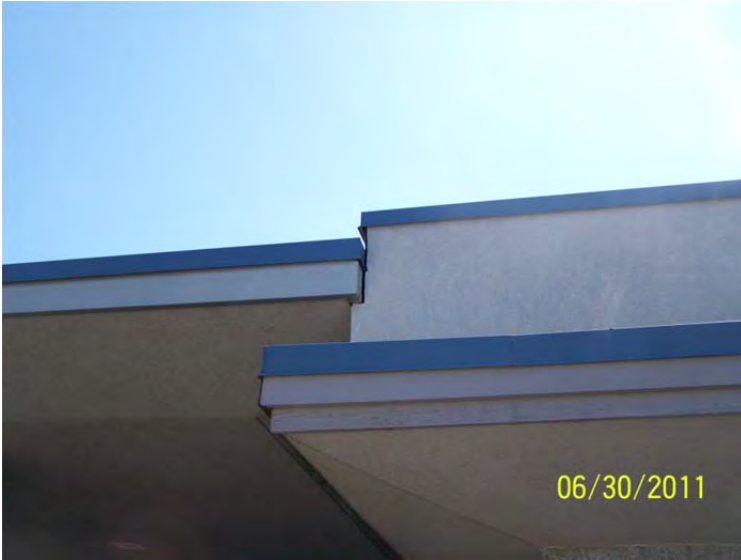
S-9: Separation in overhang roof at building parapet
