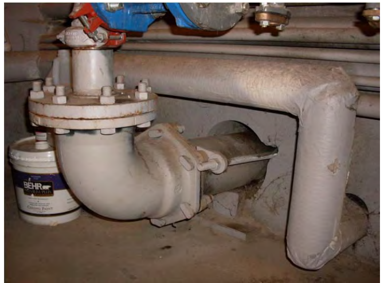
M-41: Fire sprinkler service entrance transition
