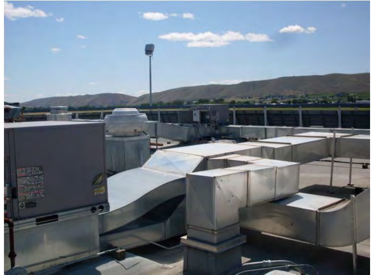
M-18: Typical galvanized steel rooftop ductwork
