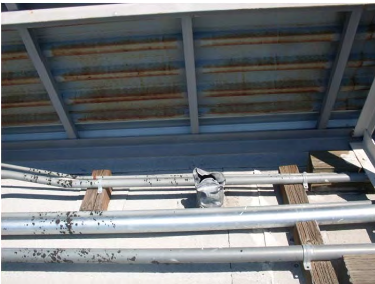
*M-24: Failing support blocks –crushed vent flashing
