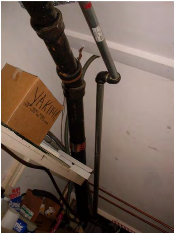
M-36: Cast iron hub and spigot waste piping
