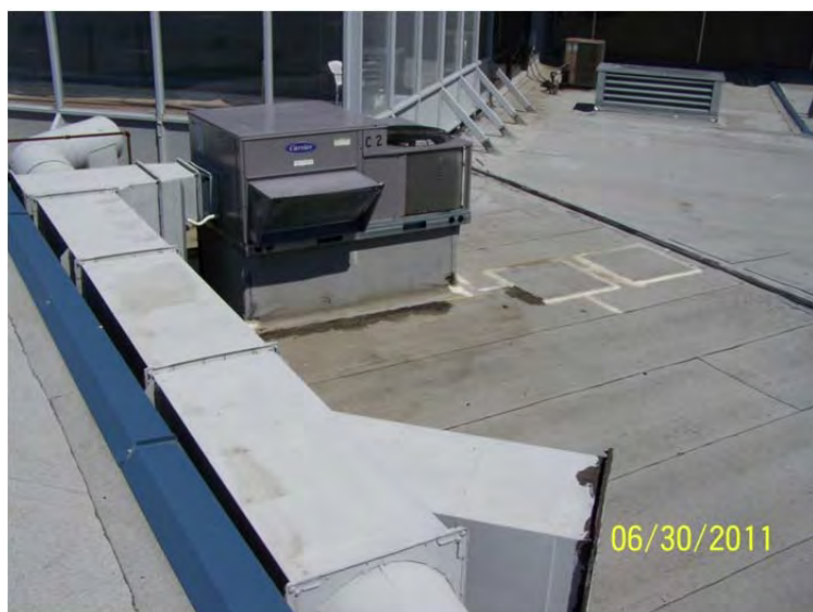
S-3: Evidence of ponding at roof
