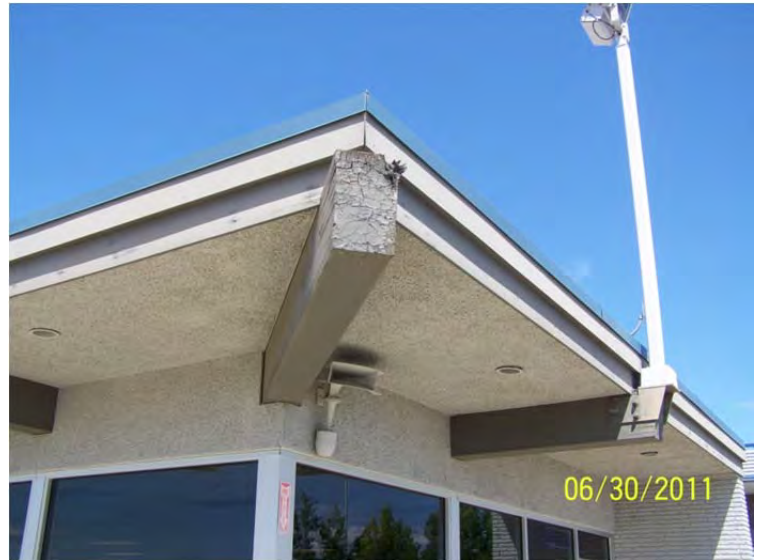
S-6: Water damage at end of exposed roof beam
