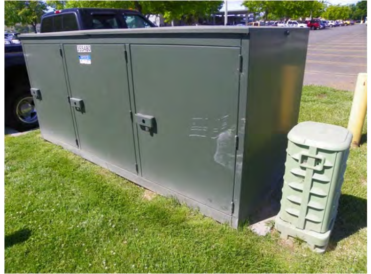
E-14: Utility primary switch and telephone pedestal
