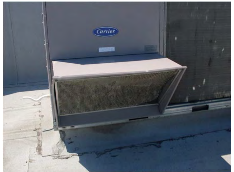
M-12: Gravity relief integral to rooftop unit
