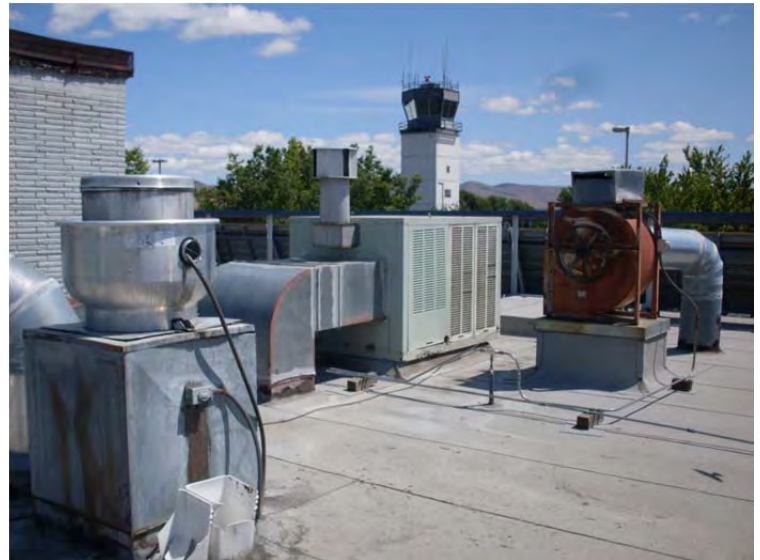
M-22: Kitchen grease hood exhaust fan
