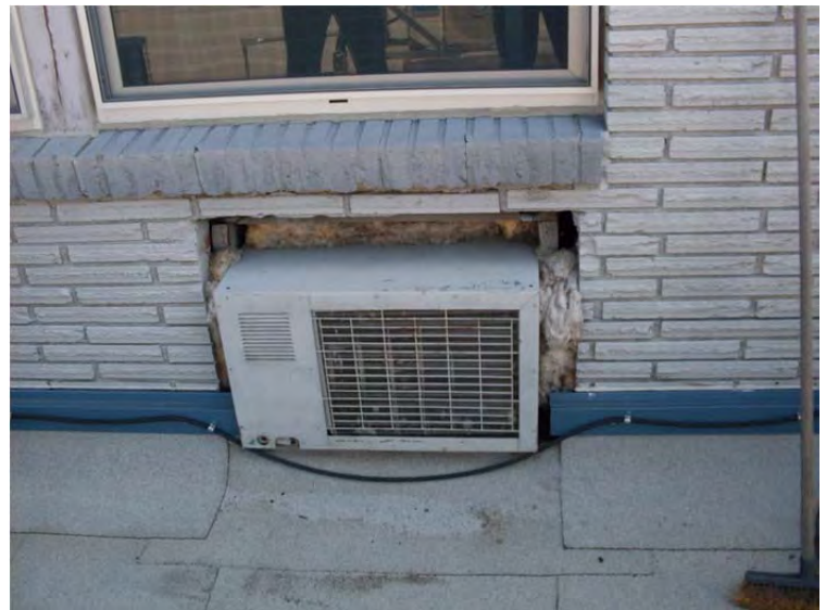
M-25: Through-wall AC unit
