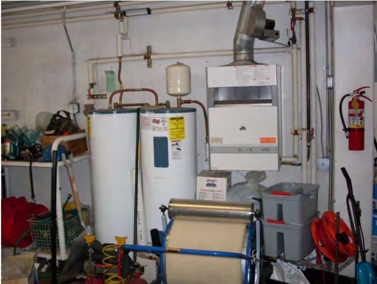
M-50: Gas instantaneous domestic water heater.
