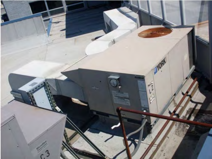
M-13: Typical rooftop ductwork
