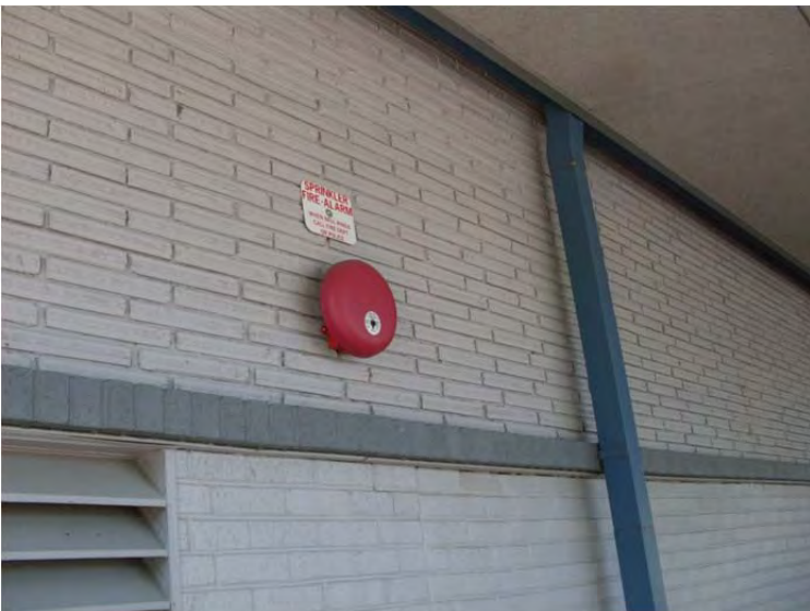
M-3: Electric fire alarm gong at front drive
