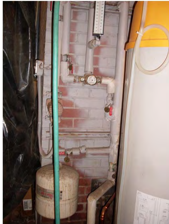
M-45: Domestic water thermostatic mixing valve
