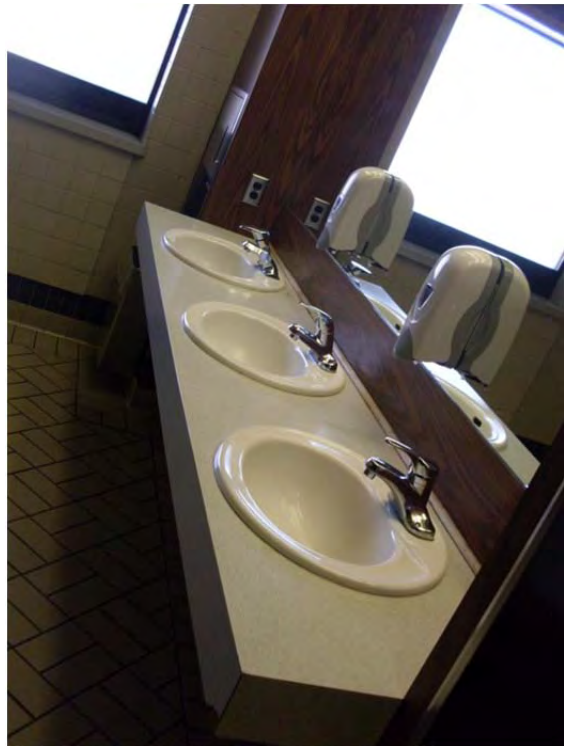
M-27: Renovated self-rimming lavatories/mixing faucet
