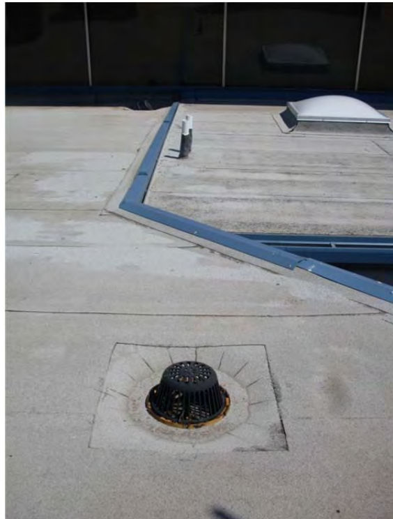
M-10: Typical roof drain
