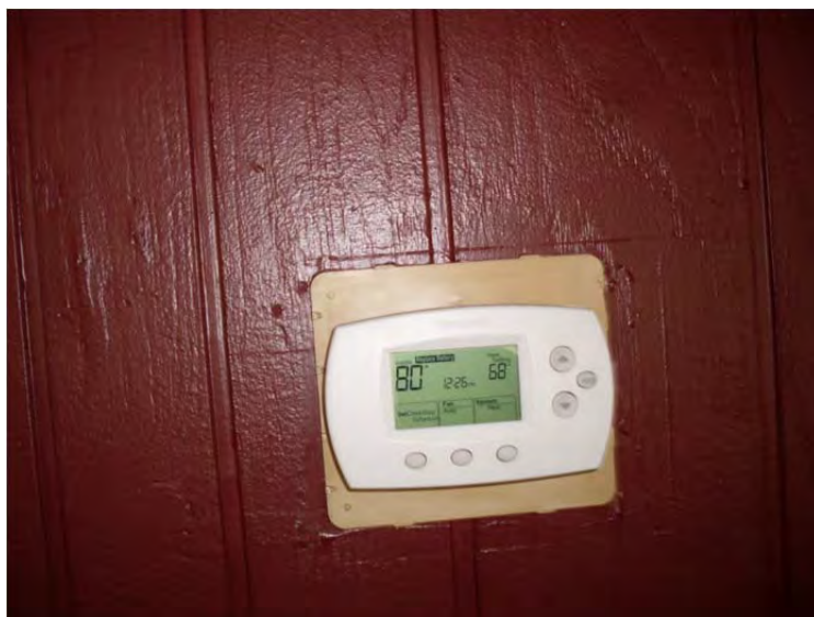
M-47: Typical newer electronic thermostat
