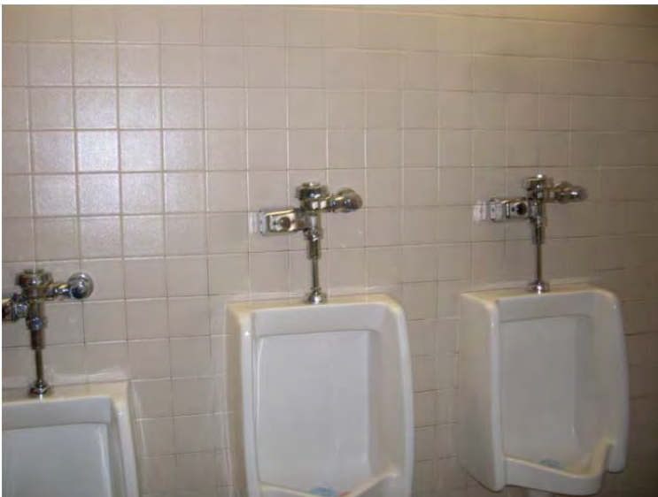
M-28: Flush valve urinals – one at ADA height
